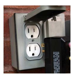
1. Plug the Ground Fault Circuit Interrupter (GFCI) into a working outlet.
